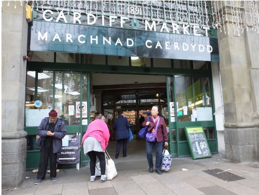
Entrance doors. Recently applied Welsh signage is a distraction from the cast iron tracery. Doors to be replaced and ironwork above refurbished.
